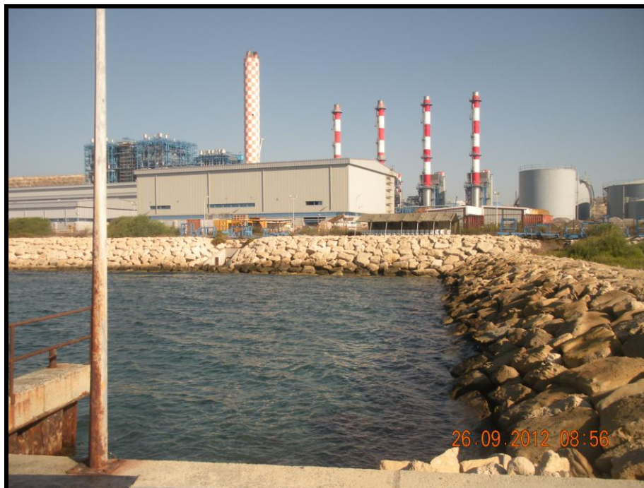
Overview of the power plant from seaside
